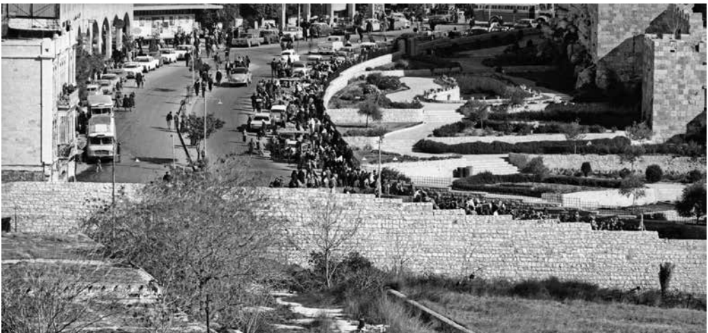
Left top: Demolition at Jaffa Gate, 1967 , photo by Ronnie Firer, online at www.tod.org.il/jerusalem50/ (accessed 18 November 2018).
